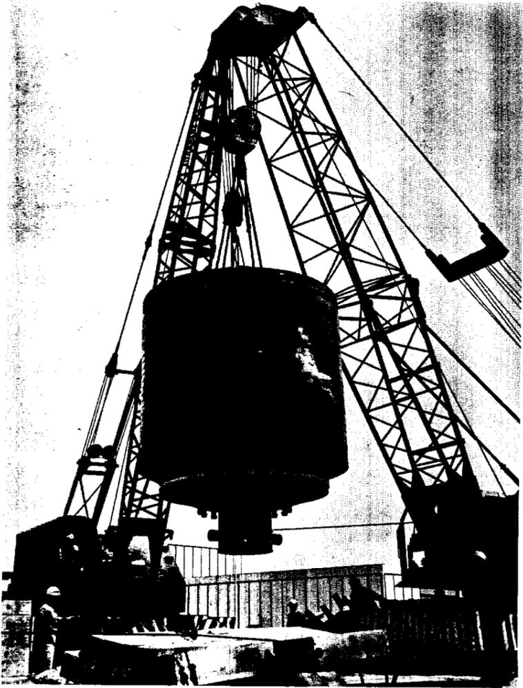
**CENTRIFUGE MOTOR PART**—Workmen use a heavy duty crane to lift the 197,000 pound rotor for the direct current drive motor which will propel the centrifuge now under construction in the Flight Acceleration Facility (Building 34). Delivery was made last week on this part of the largest DC motor ever built which develops 10,700 horsepower. The centrifuge will be capable of generating 30 g's of force on material and lower forces for personnel.
