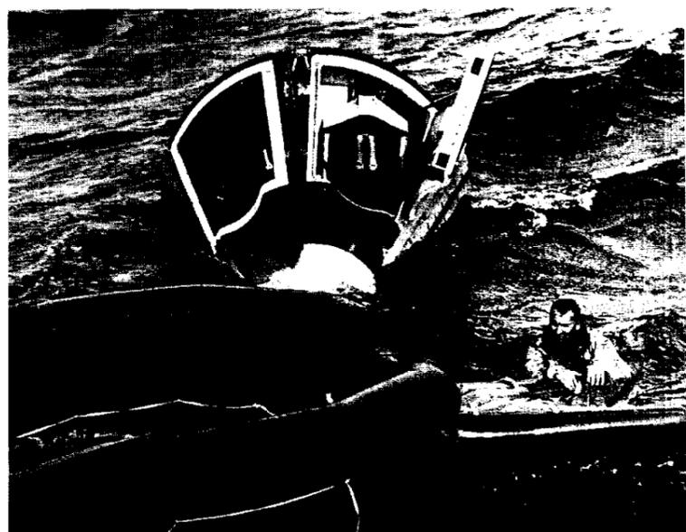
**ROUGH WATER RECOVERY**--The Rendezvous and Recovery section of a boilerplate version of the Gemini spacecraft is completely awash during rough water egress tests in the Gulf of Mexico. Astronaut James A. Lovell Jr., one of the test participants is in the water with waves running six to eight feet high.
